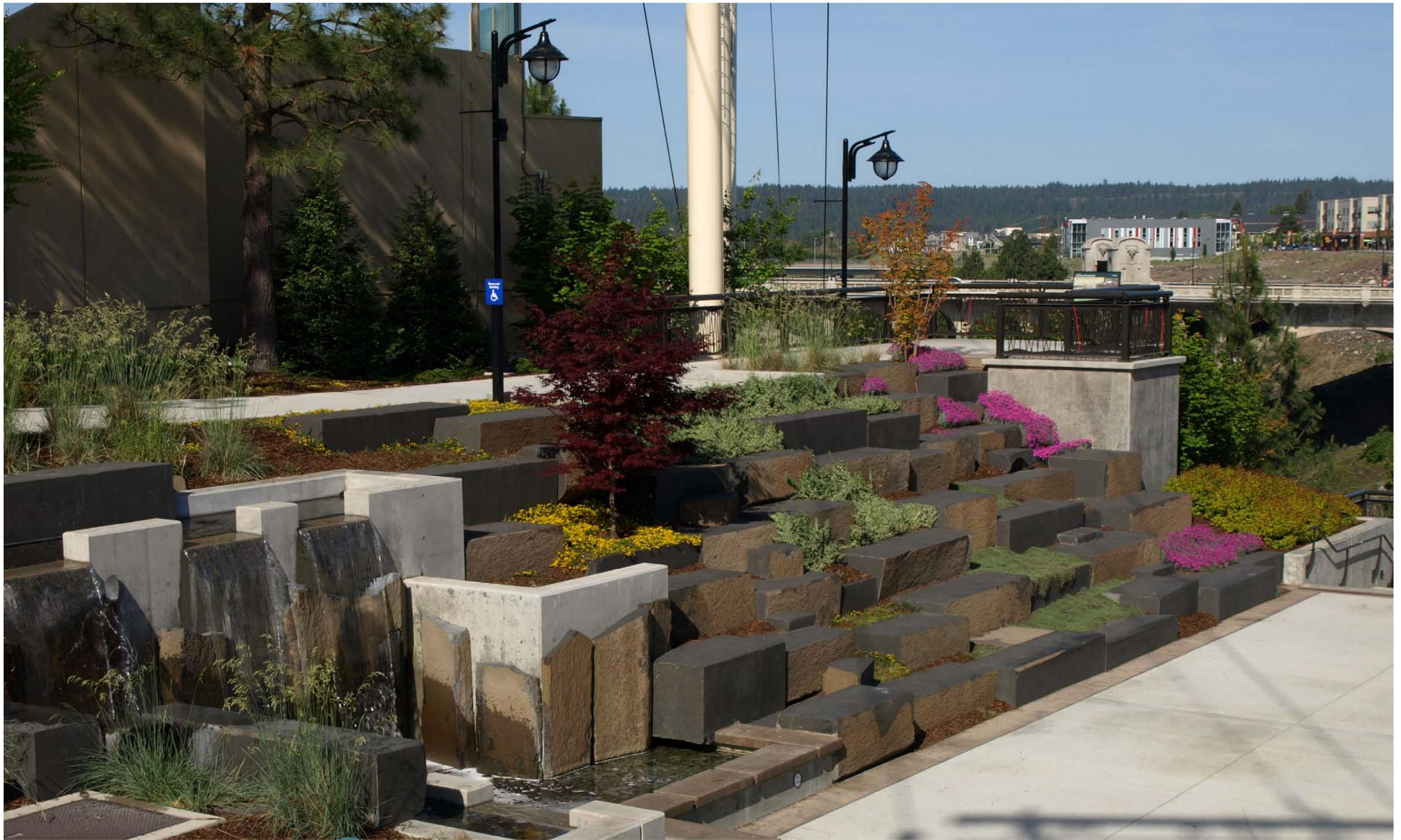
CONNECTIONS – Cut native basalt was used for amphitheater seating. Remnants from the cut stone were used to face the water feature representing the Monroe Street Dam and the native basalt river bed.
